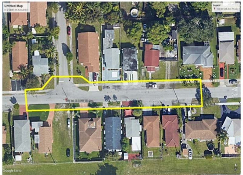
45th yr CDBG 7 th Ave and 3 rd Ct Stormwater Improvements, City of Hallandale Beach
